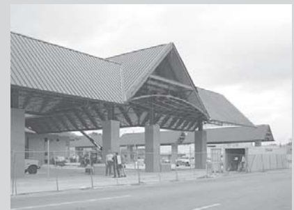
Downtown Transit Center under construction
