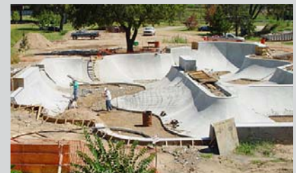
Construction is underway for Oklahoma City's first public Skatepark.
