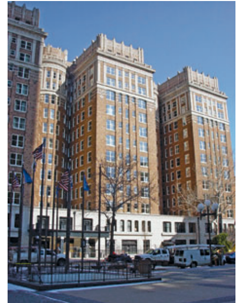
After being shuttered for two decades, the newly renovated Skirvin Hotel opened last month. The hotel is considered a great example of thoughtful planning espoused by the Urban Land Institute.
