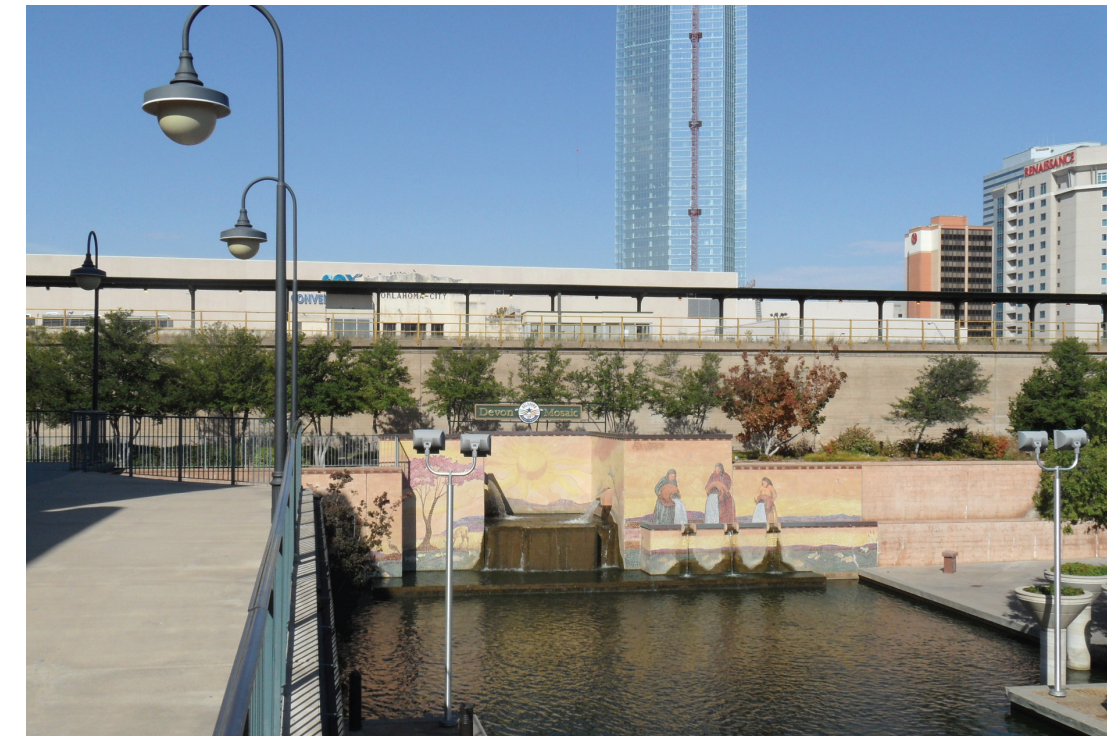
Existing Conditions @ Bricktown West Canal - Figure 9.7
