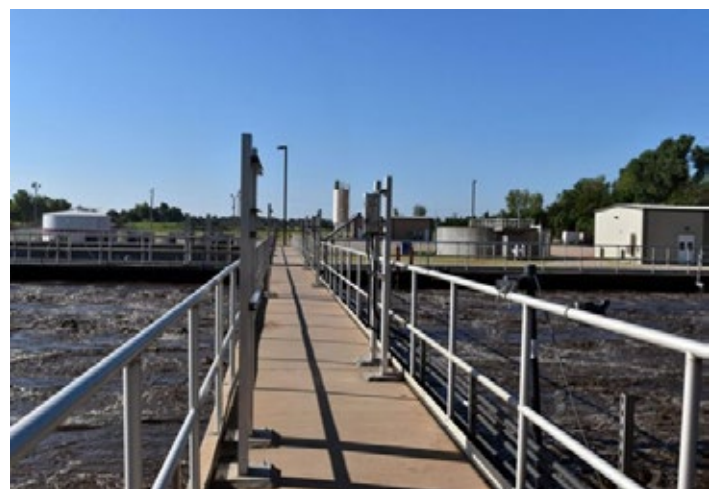
Figure 8: New Water Reclamation Facility in Mustang 16
